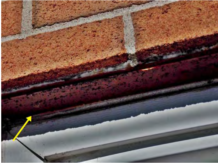
A close-up of rust on a window lintel.
