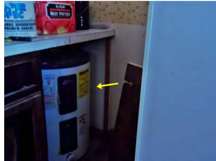
Each unit has its own electric-heated DHW tank.
