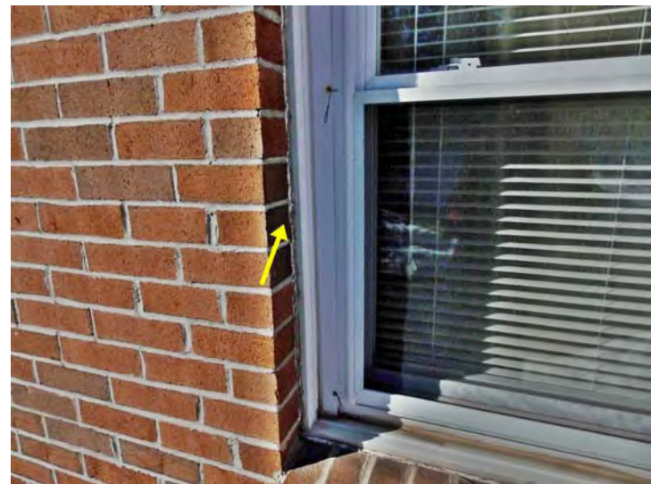
Caulking around windows is dried out and cracked.
