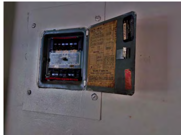
There are units that still have original Federal Pacific (Stab-Lok) circuit breaker panels, which have a history of failing to fully react to an electric overload condition.
