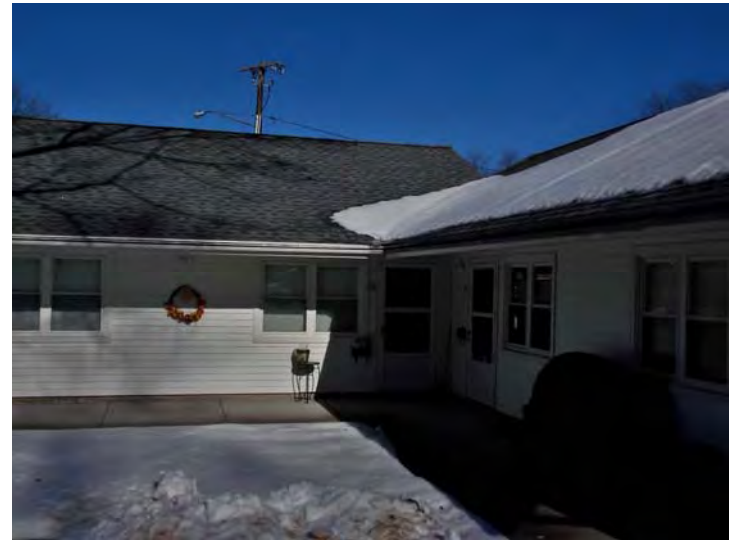
Roofs have been recently covered with architectural asphalt shingles.
