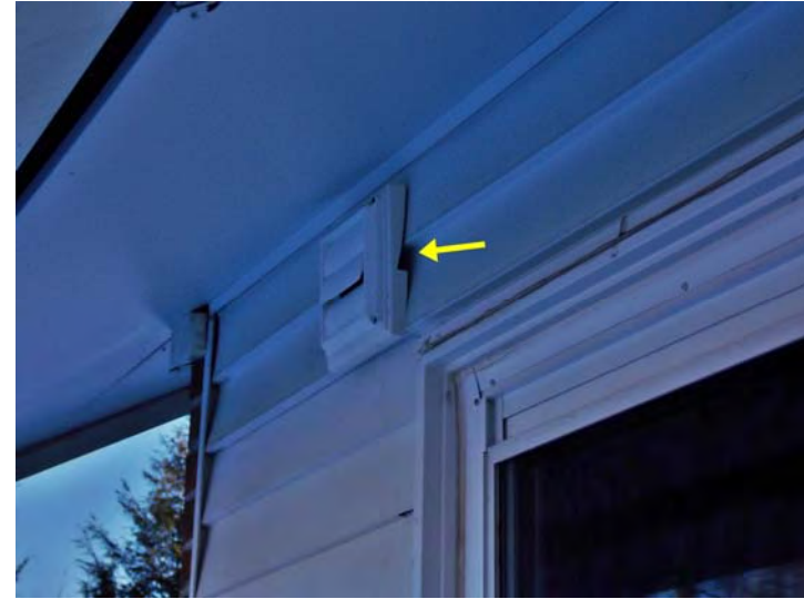
The mounting of the bathroom exhaust cover provides the opportunity for possible debris collection or insect nesting.
