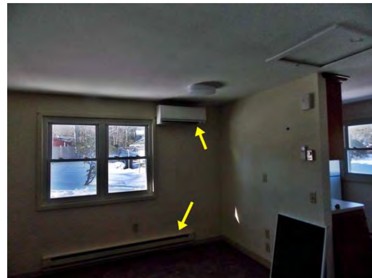
Recently installed heat pumps (upper arrow) provide heating and cooling. The electric baseboard (lower arrow) is original and can provide additional heat.
