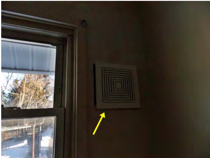
Bathrooms have been upgraded with wall-mounted exhaust fans.
