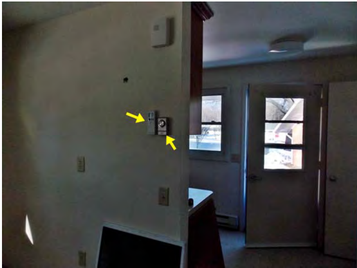
The heat pump control (on left) and the electric baseboard thermostat (on right).
