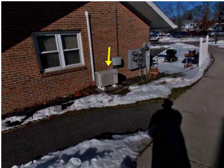
One of the air-cooled heat pump condensers.
