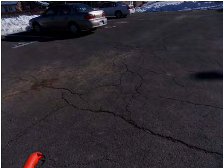
A section of cracked asphalt paving.
